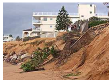
Erosion at Collaroy
